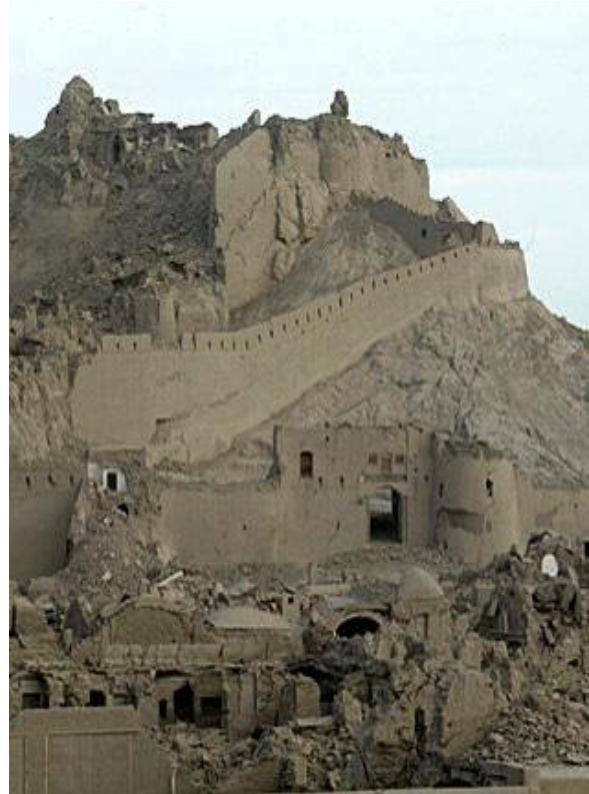
5. Iran. Bam after the violent 2003 earthquake.
